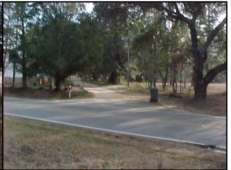
Looking at site entrance from Trotter Rd
